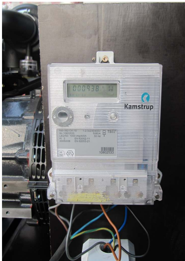
The power consumed by the load was measured by an accurate 3phase electrical meter. On the photo the load was 9,38kW – close to full load.
