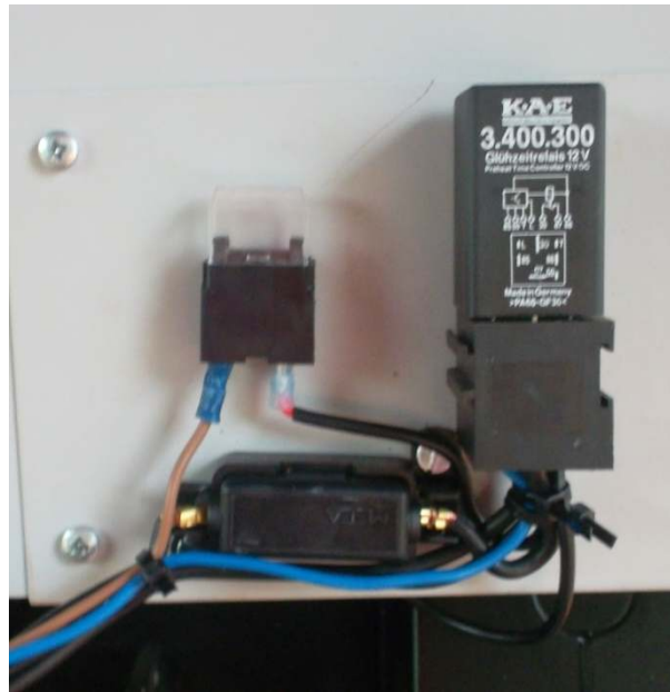
New glow plug controller(relay) installed on the read side of the genset controller.
