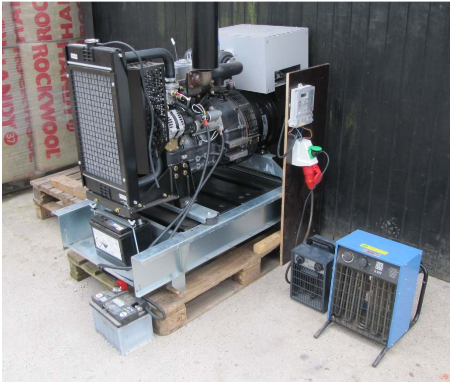
Load test with electrical air heaters and measurement of the consumed power.
