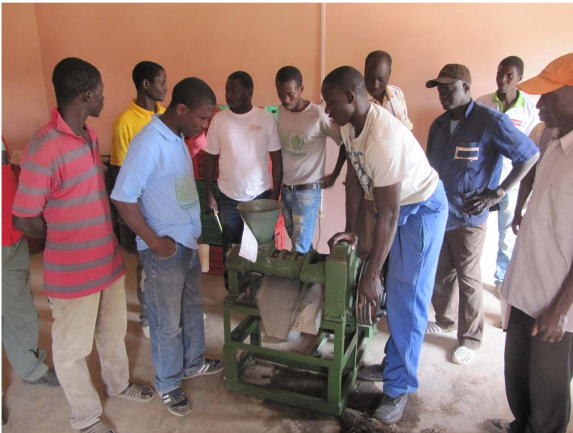
Checking the oil expeller and agree how to install it. We had to build a frame with supports to lift the expeller up from the ground in order to build an oil sedimentation system with natural flow by gravity.
