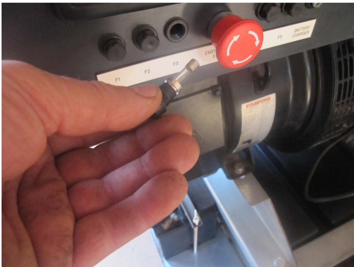
Found that the error was caused by one of fuses which had become loose.
