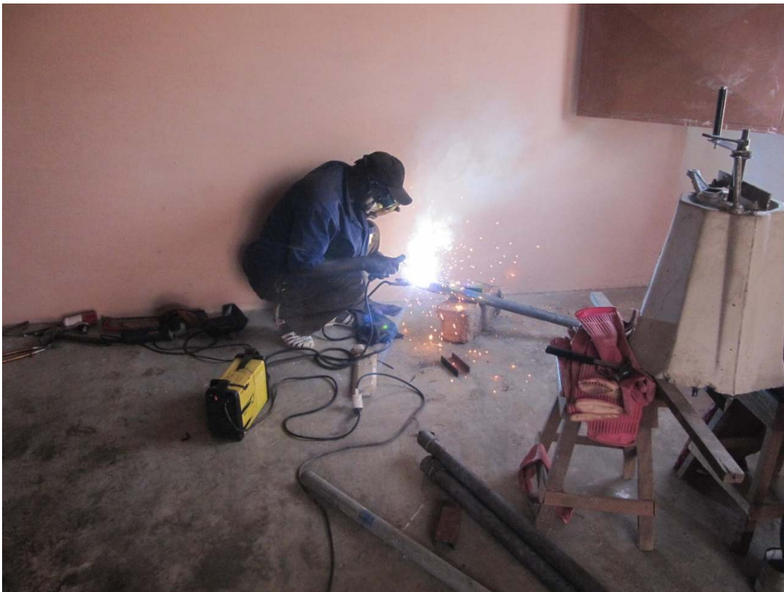
Welding legs to the support frame
