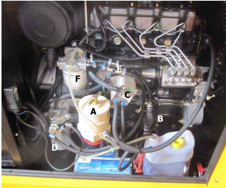
The main components for the conversion of the Perkins Genset.
